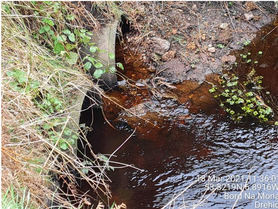
Photo 2 Current Outflow Pipes from Old Settlement Ponds
